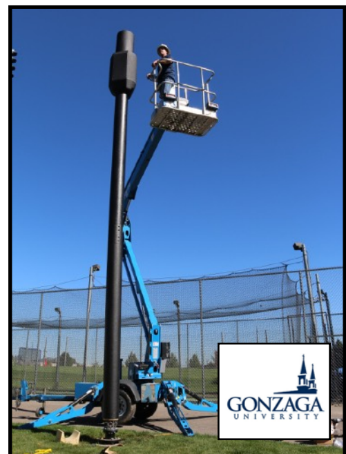
The composite towers are easily handled with minimal equipment
